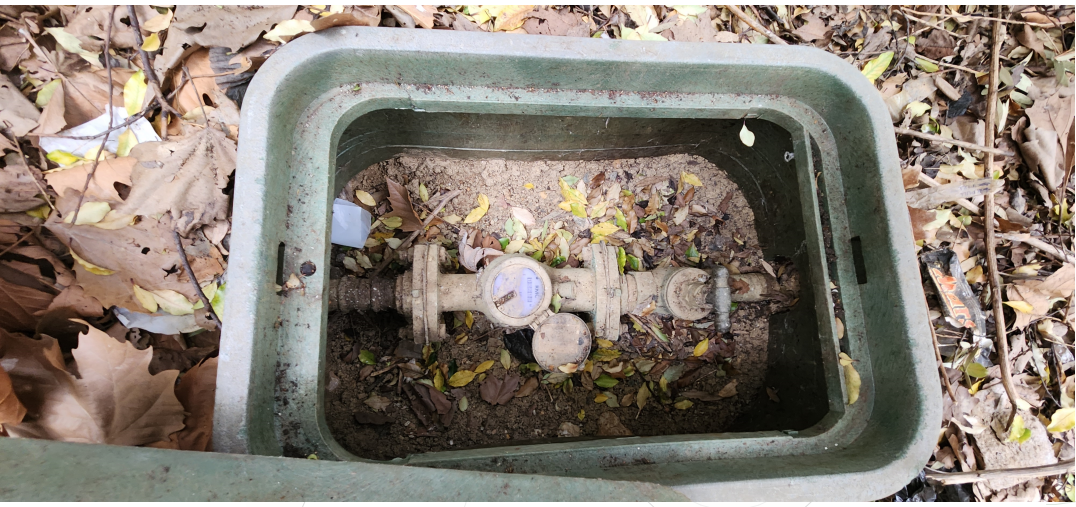
Photo 1: Existing site authority master water meter.
